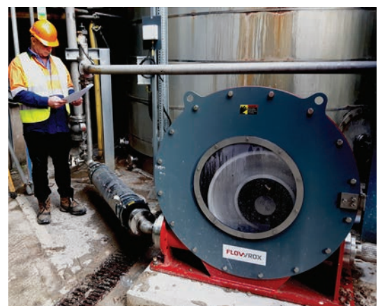
Flowrox LPP-T pump with 80 mm Expulse stabilizing the flow in a filter feed application.
